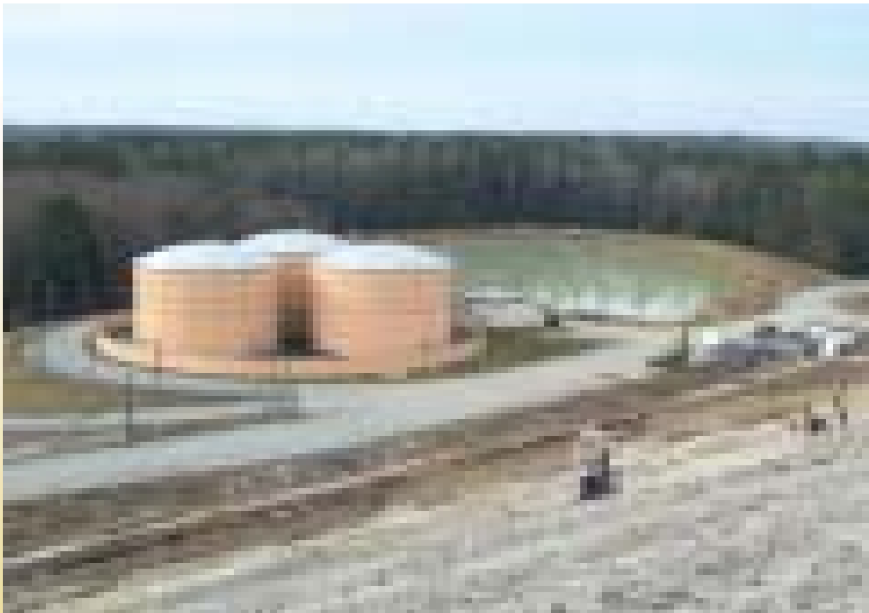
An expanded leachate containment system using glass-lined steel tanks. Each tank has 330,000 gallon (about 1.3 mega litres) capacity. In the foreground are landfill gas headers, connected to landfill gas wells, in a closed landfill cell. Jones Cross Roads Landfill Site, Delaware, USA.
